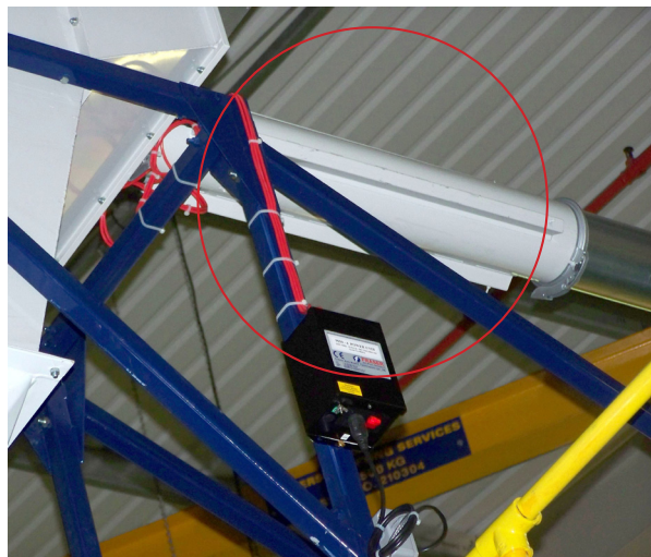
6000 lontube mounted before the separator.
